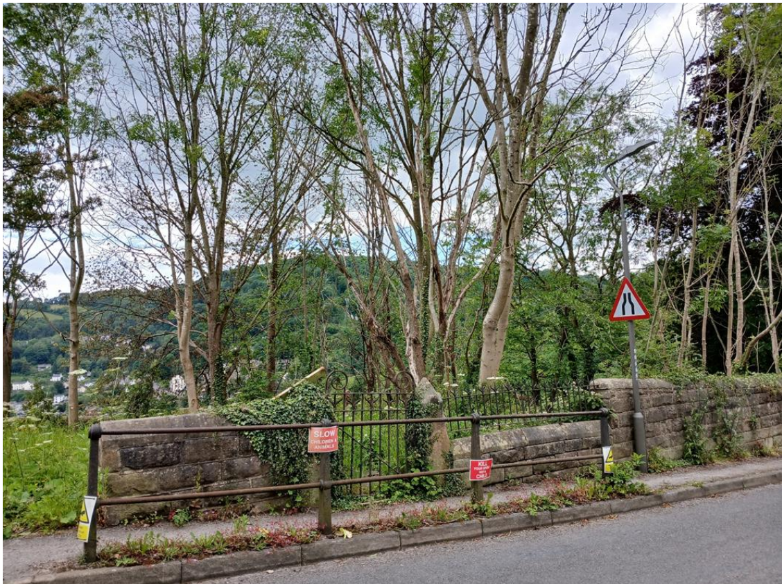
[Photo 1: Existing pedestrian metal gate, railings and boundary wall along eastern boundary]
