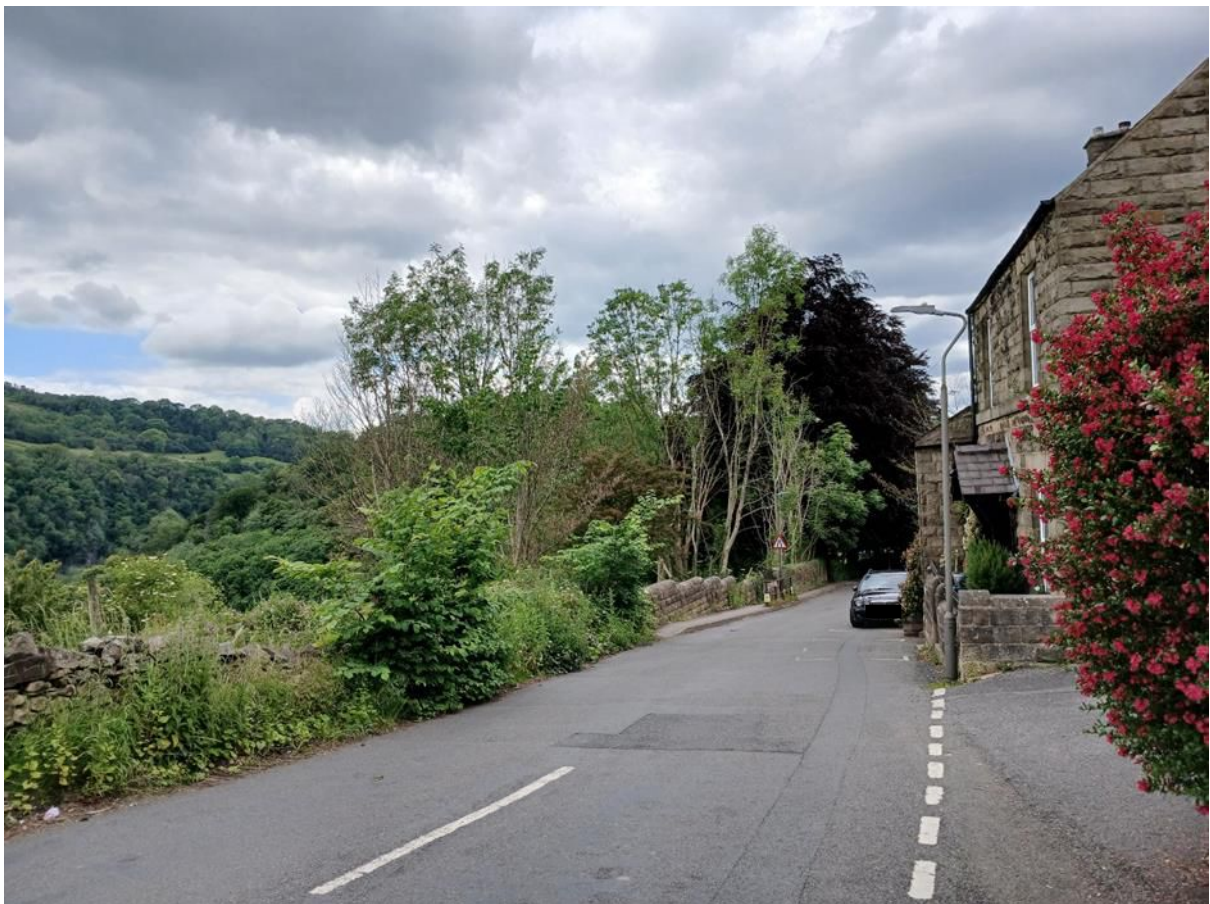
[Photo 4: Looking north towards site from Starkholmes Road]
