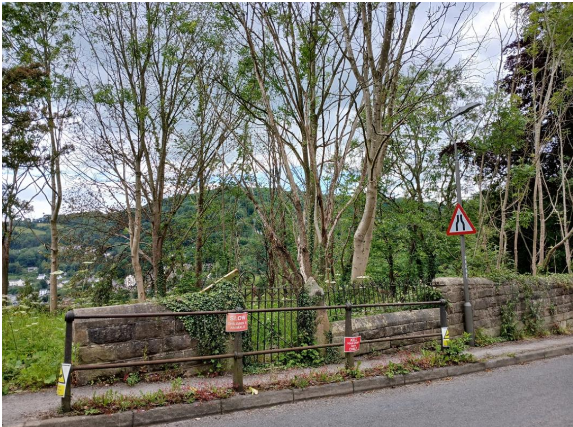
[Photo 1: Existing pedestrian metal gate, railings and boundary wall along eastern boundary]
